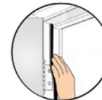
**4 APPLYING WEATHER STRIPPING** - Peel back the self-adhesive foam. Apply one continuous strip of material snugly along each side. Make sure the weather stripping meets tightly at the corners and is pressed firmly onto the door and door jamb. The material should compress tightly between the door and door jamb, without making it difficult to shut.
